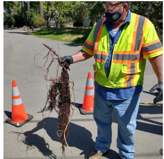
Figure C - Root intrusion pulled from the collection system
