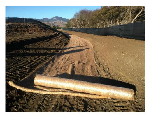
Liner work is complete along the north side of the basin. Liner work is continuing on swale to the east of the impoundment basin.
