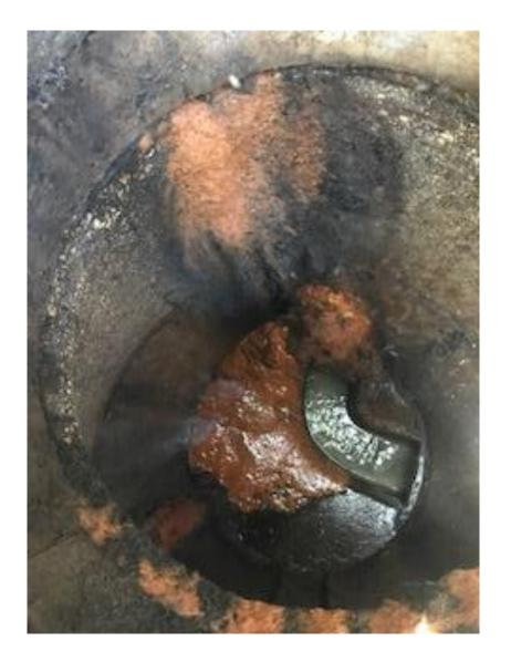
This manhole is one of the manhole we have identified as having problems. The manhole is leaking water even during the dry season. The cost to repair the leak is \$6,000 and we have several just like this one. The leak is coming from the connection 4 feet up from the bottom. This is not something that replacing the lid can fix.
