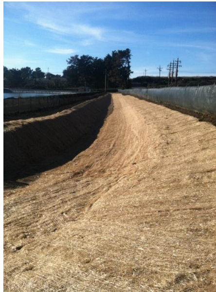
12/1/2017 Lined Swale along North Side of Impoundment
