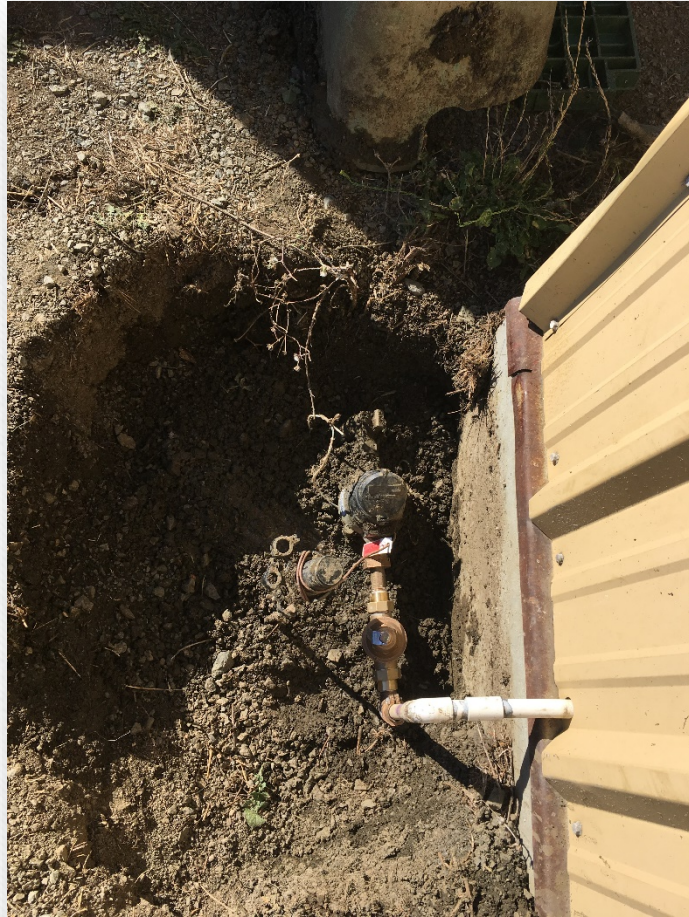
This pressure regulator is located at SS3. The water that goes through the regulator is for the chlorine analyzer and the turbidimeter for the entire SS wellfield.
