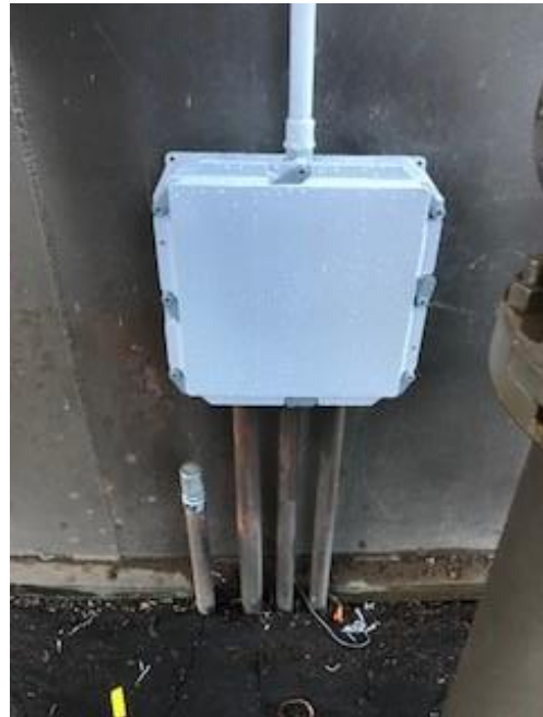
Figure 3 Rusted electrical pull box
